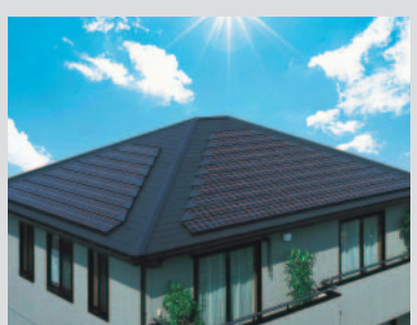
Residential photovoltaic generating systems
