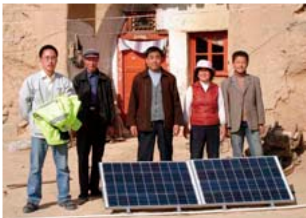
Solar power generation system donated to un-electrified village in Gansu Province, China in April 2006
