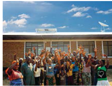
Solar modules installed at a school (Tanzania)
