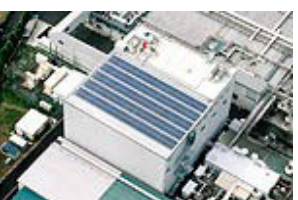
■ Kagoshima Hayato Plant (40kW) (introduced in FY2006)
