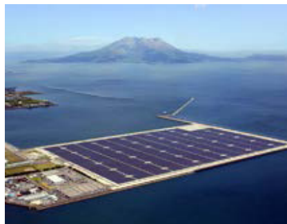
Kagoshima Nanatsujima Mega Solar Power Plant where Kagoshima Nanatsujima Solar Science Museum is located
