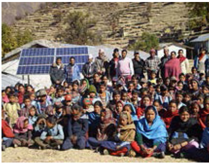
Solar modules installed at a school (Nepal)
