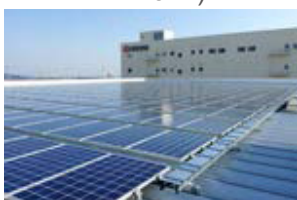
■ Shiga Yohkaichi Plant (1,137kW) (introduced in FY2006, expanded in FY2011, FY2012, FY2013, FY2014)
