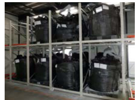
Sludge drying equipment
