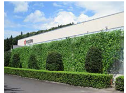
Green Curtains (Fukushima Tanagura Plant)
