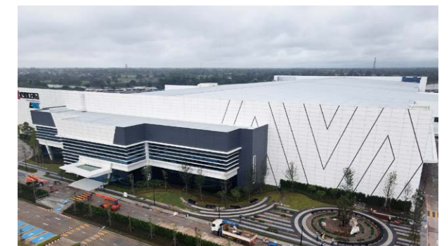
The new KYOCERA AVX Thailand Plant
