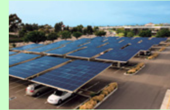
Installation ex; Parking lot
