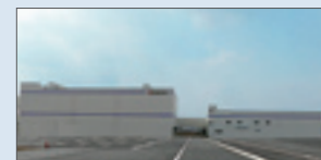
Kyocera Mita Corp. Tamaki Plant Plant No. 4, Chemical Product Development Center
