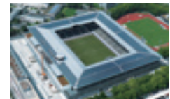
Solar Power Generation System
