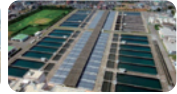
Asaka Water Purification Plant, Saitama Prefecture
