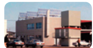
The first grid-connected system in Japan installed on a general facility in Kitami City, Hokkaido, in 1991 (The solar power system is connected with the power company system)
