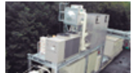
Freezing Concentration & Ice Thermal Storage System
