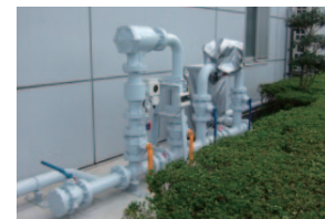
Newly installed gas piping
