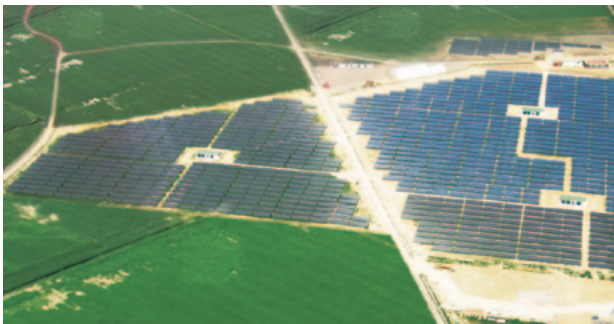
Solar power plant in Cigliano, Piedmont, Italy
