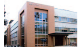
Inamori Academy building
