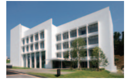
Inamori Foundation Memorial Hall housing the Inamori Frontier Research Center
