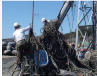
Restoration work underway
