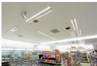
Convenience store using Kyocera's LED lighting
